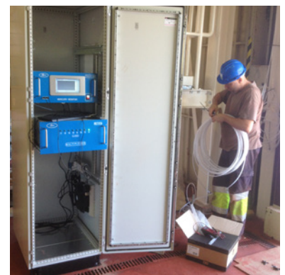
Indoor mercury monitoring at the Hg treatment plant in Europe
